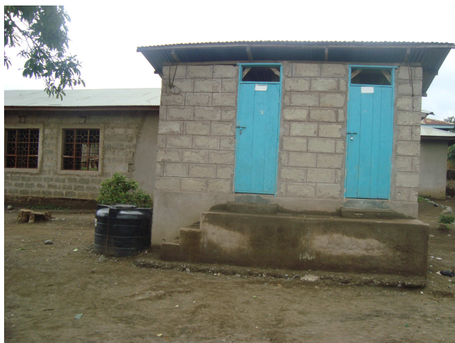
Fig. 5: Concrete block four vaults UDDT in Daraja II primary school, the plastic tank for urine collection can be seen on the left side of the toilet.
